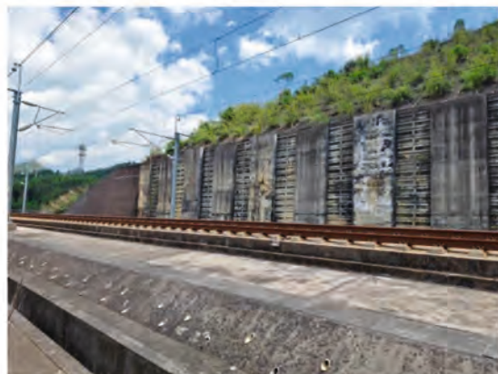
K763+690 坡面溜坍边坡防护
